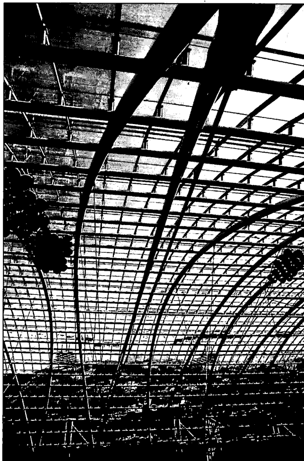
Figure 7.5 Chur Station, Switzerland
